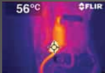
What a thermal imaging camera sees.
