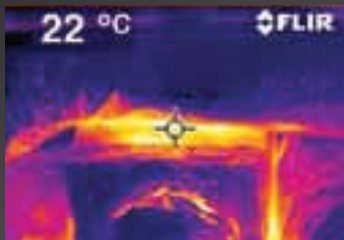
What a thermal imaging camera sees.
