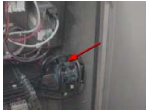
Thermal and Digital Image showing poor connection on Main Isolator Switch
