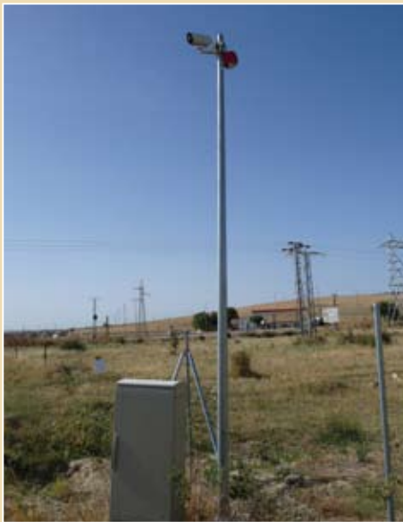
An observation point with a thermal imaging camera and a light/sound beacon. The electrical cabinet contains a FLIR Systems Mini Server (1) a FLIR Systems I/O box (2) and an Ethernet/ Fiber optics converter (3).
